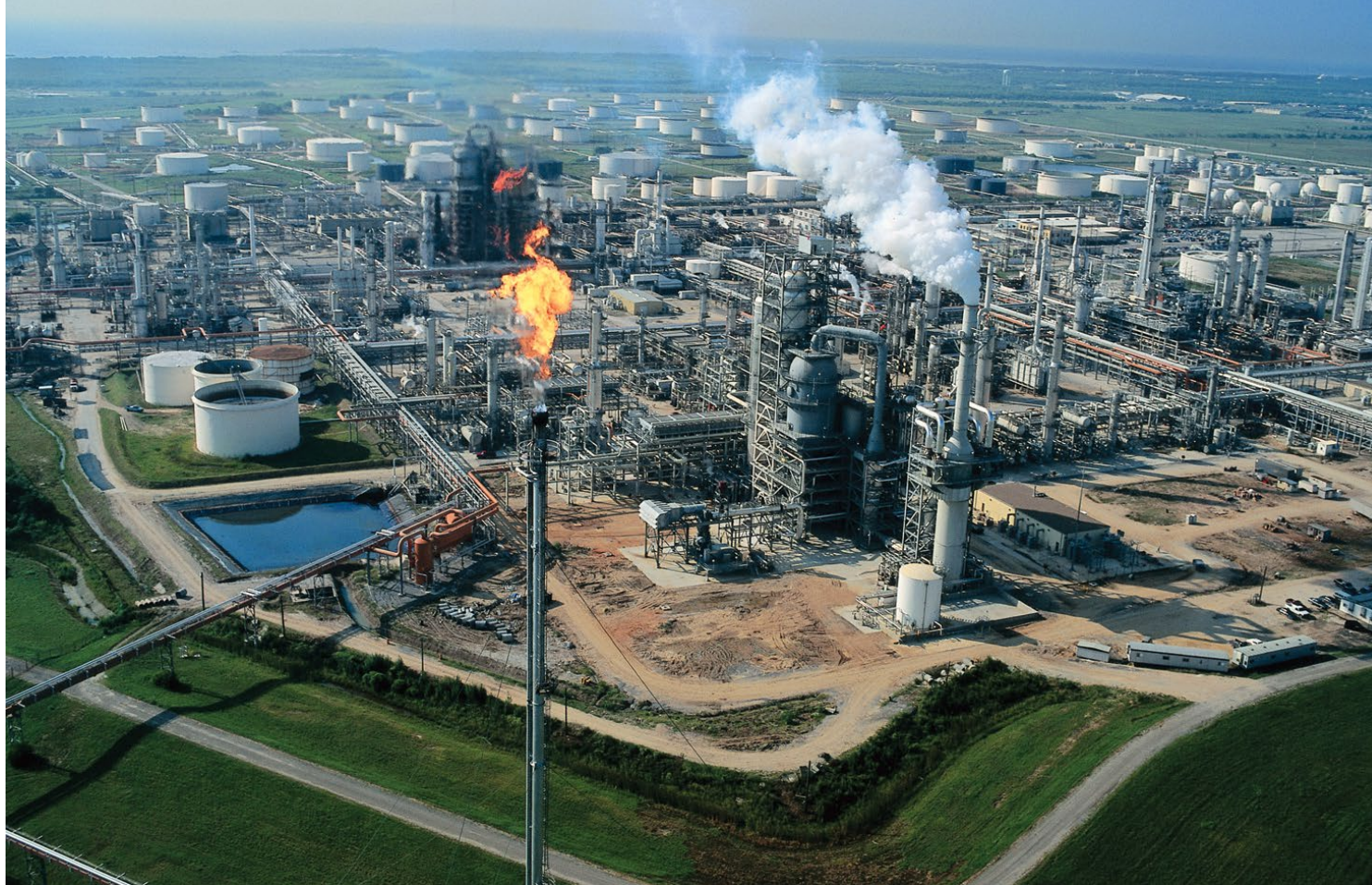
Photo of a crude oil refinery showing the tall distillation towers.
